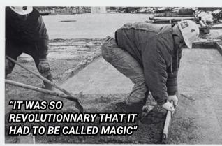
In 1984, Quebec City concrete finisher, Roger Rouillard, transformed the concrete industry. He invented the first handheld vibratory screed that floated on concrete.
